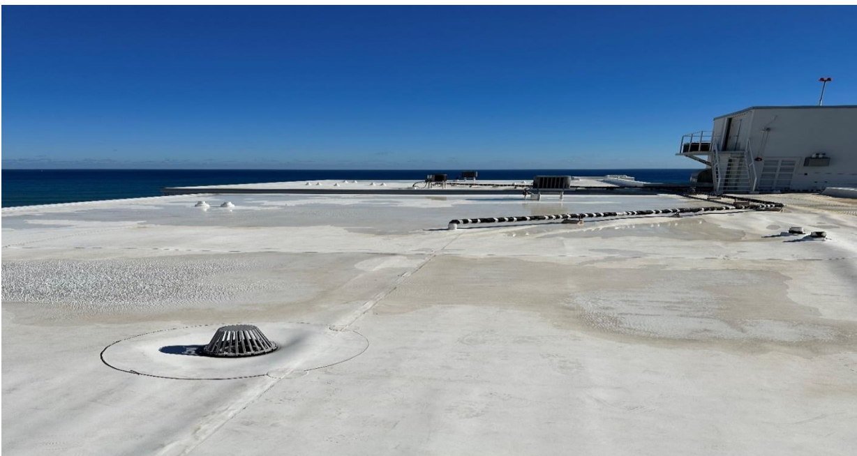
Photo 5: West Tower Roof, Looking East
