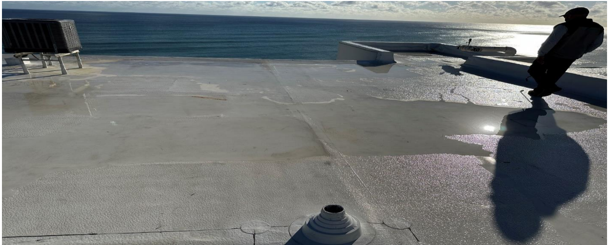
Photo 6: East Tower Roof, Looking East
