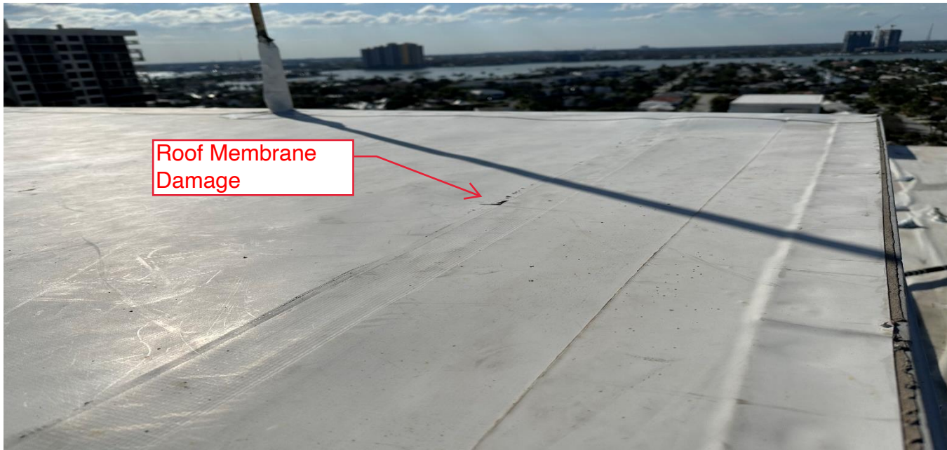
Photo 8: Elevator Tower Roof, Looking West
