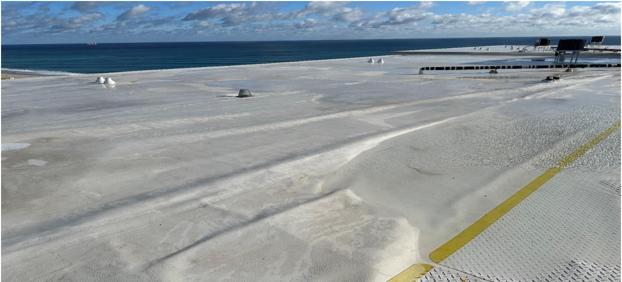
Photo 4: West Tower Roof, Looking Northeast.
