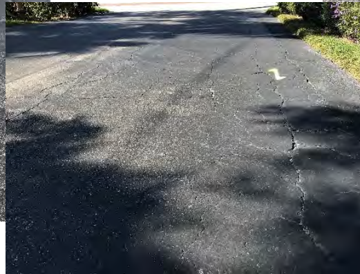
Parking Area Asphalt
