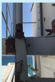
Roof stairs welding
